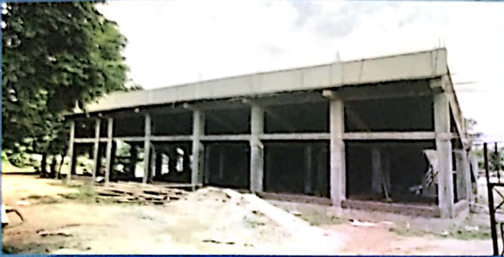
Outdoor Pavillion undergoing construction
